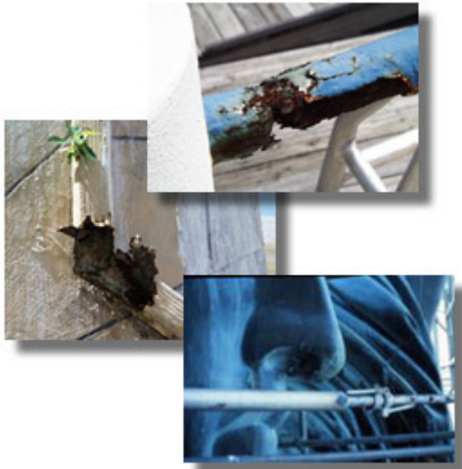
Corrosion on the Nose of the Statue of Liberty
