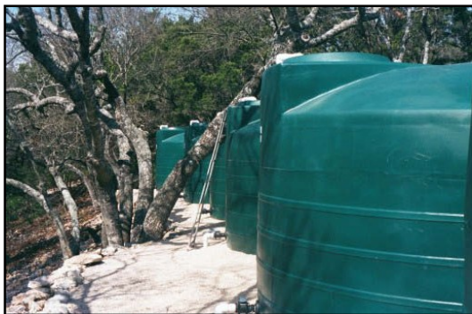
Figure 2-6. Low-profile 5,000-gallon polypropylene tanks
