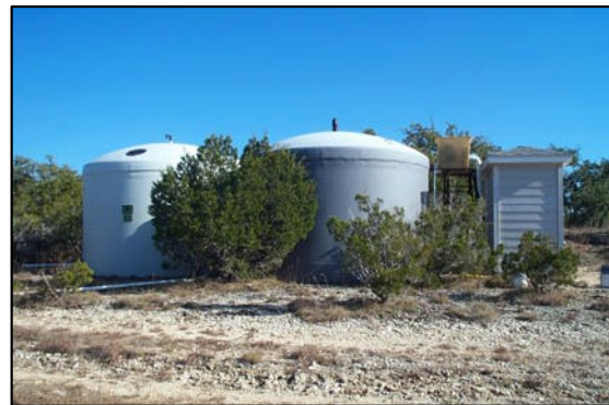
Figure 2-5. Two 10,000-gallon fiberglass tanks
