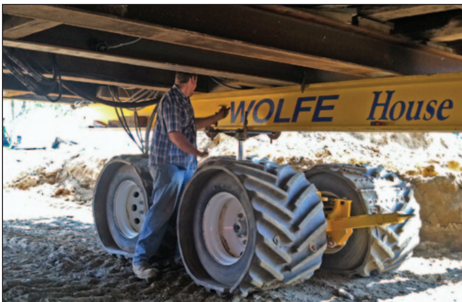
Figure 5R-11. Trailer wheel sets are placed beneath the lifting beams (photo courtesy of Wolfe House Movers)
