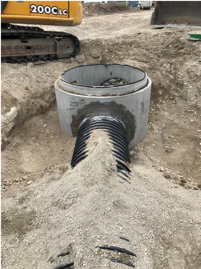
Figure 38 – Installed Steel Reinforced Corrugated HDPE
