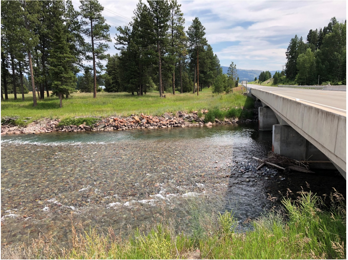
Figure 11 – Riprap upstream from a bridge.
