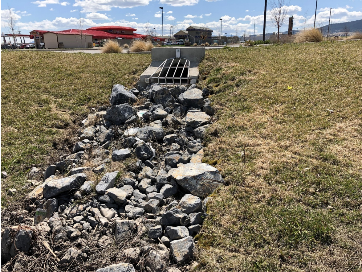
Figure 19 – Culvert outlet with riprap protection
