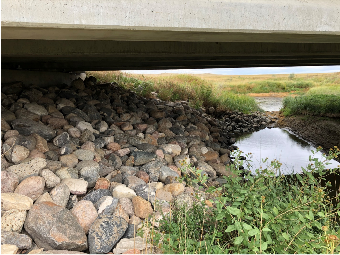
Figure 13 – Riprap protecting a bridge abutment
