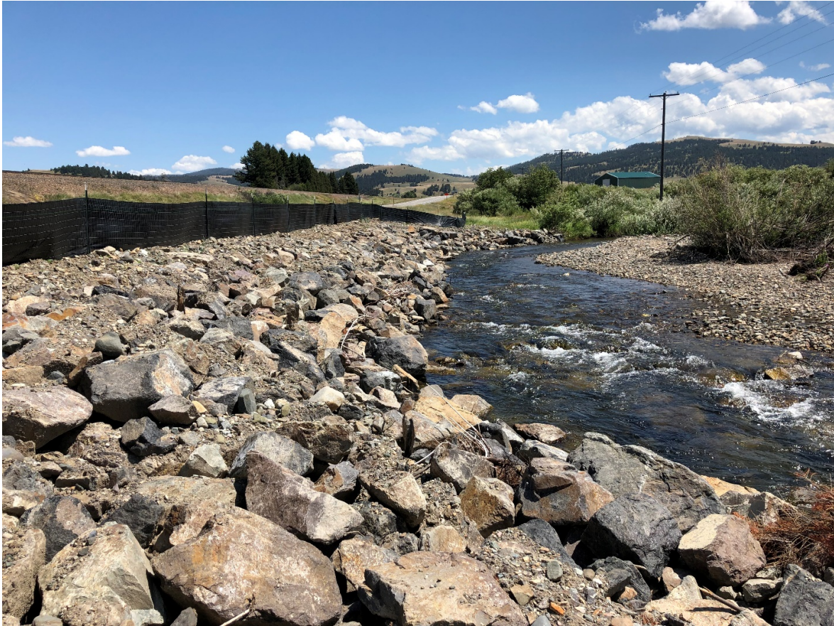
Figure 9 – Riprap protecting a highway embankment adjacent to a stream
