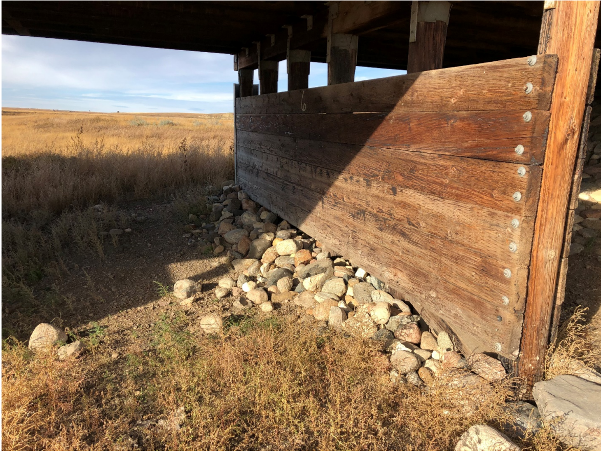
Figure 14 – Riprap around bridge pilings
