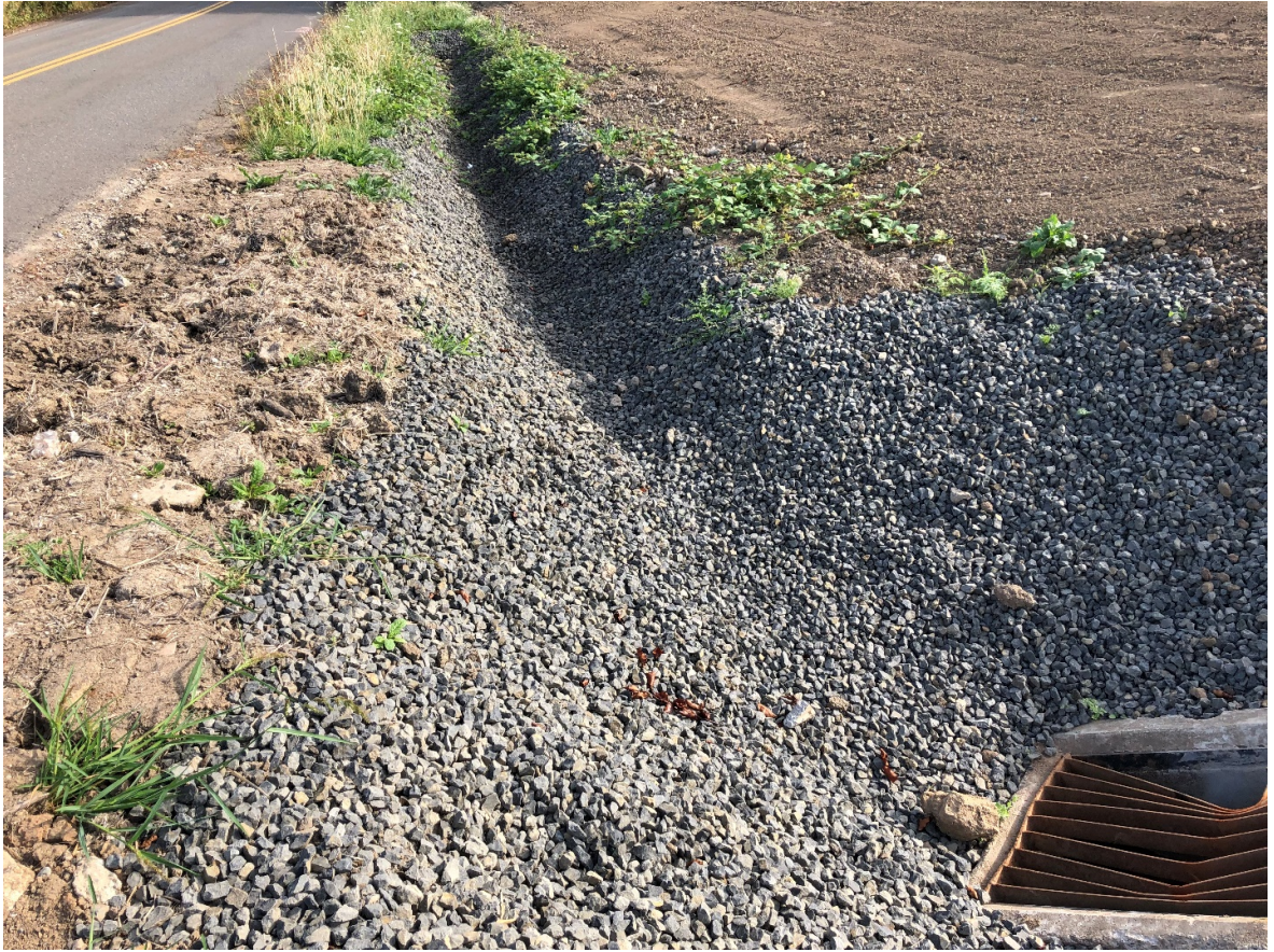
Figure 16 – Channel with fine gravel for erosion protection
