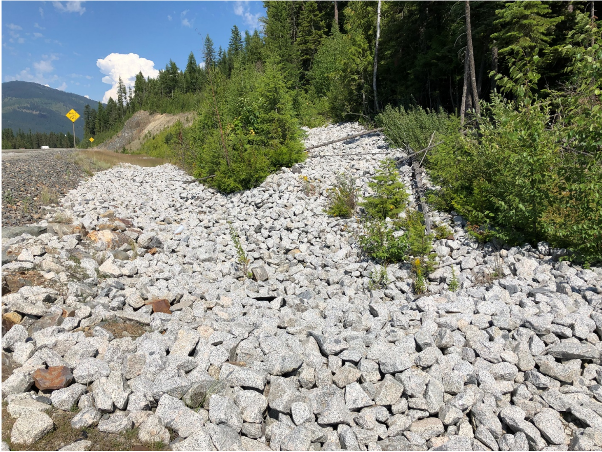
Figure 17 – Channel with riprap for erosion protection
