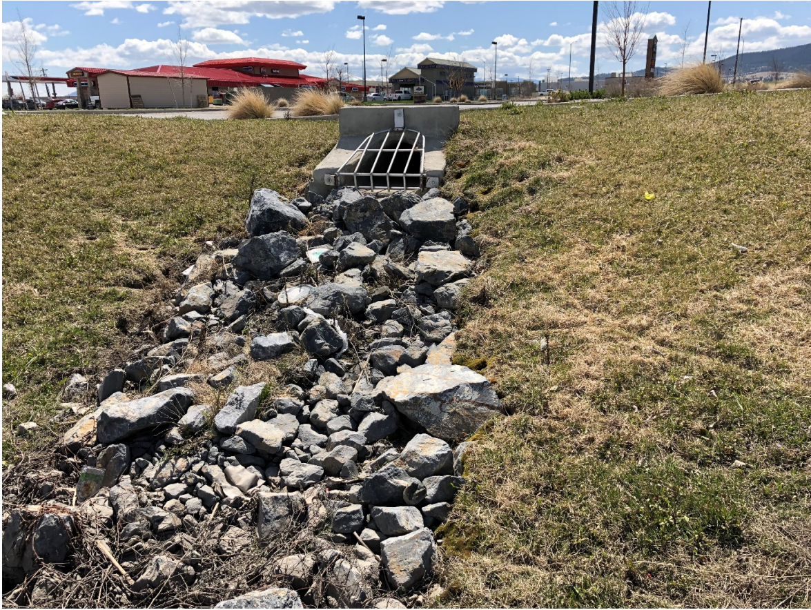
Figure 7 – Riprap at downstream end of pipe
