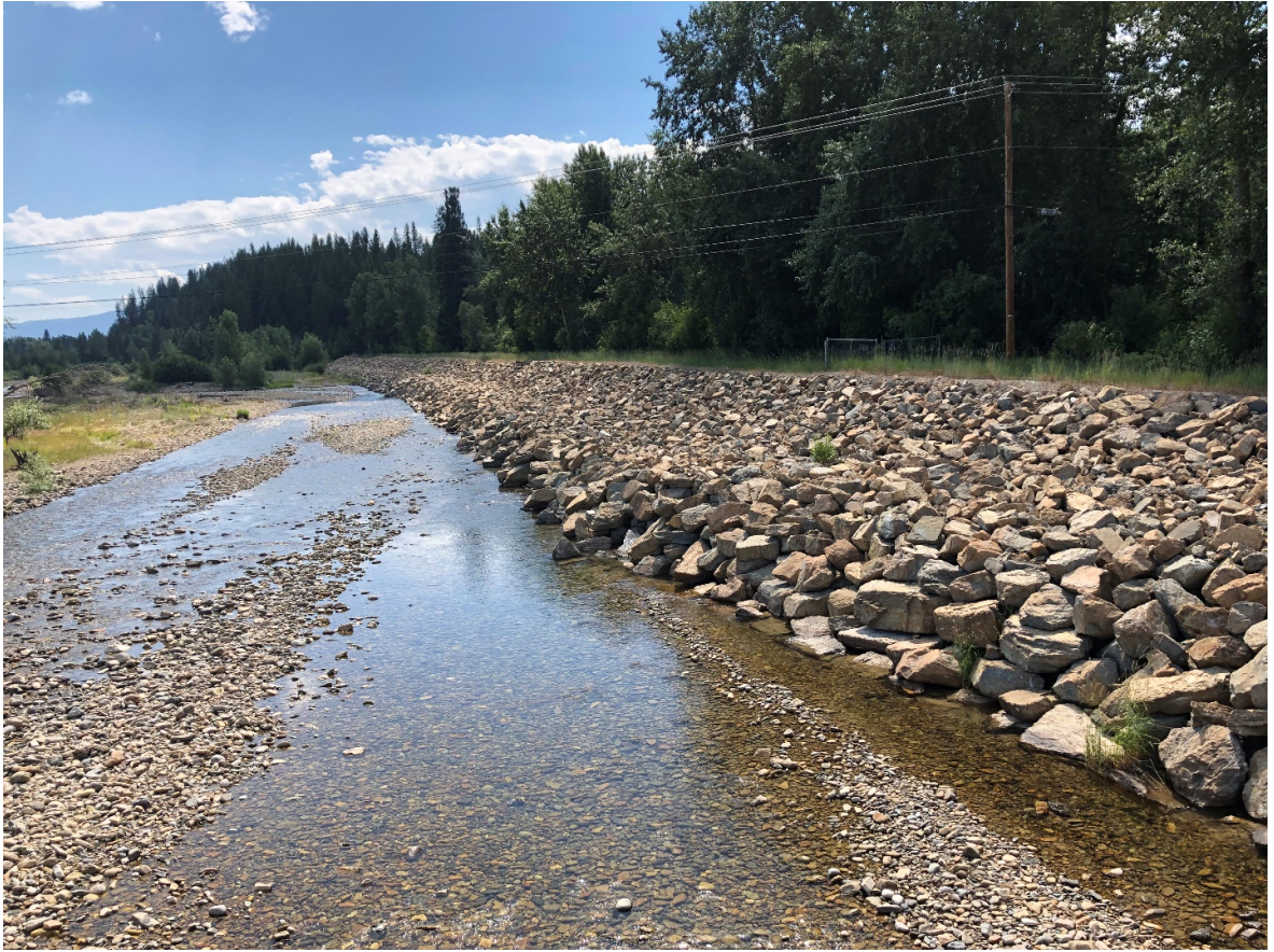
Figure 12 – Riprap guide bank upstream from a bridge
