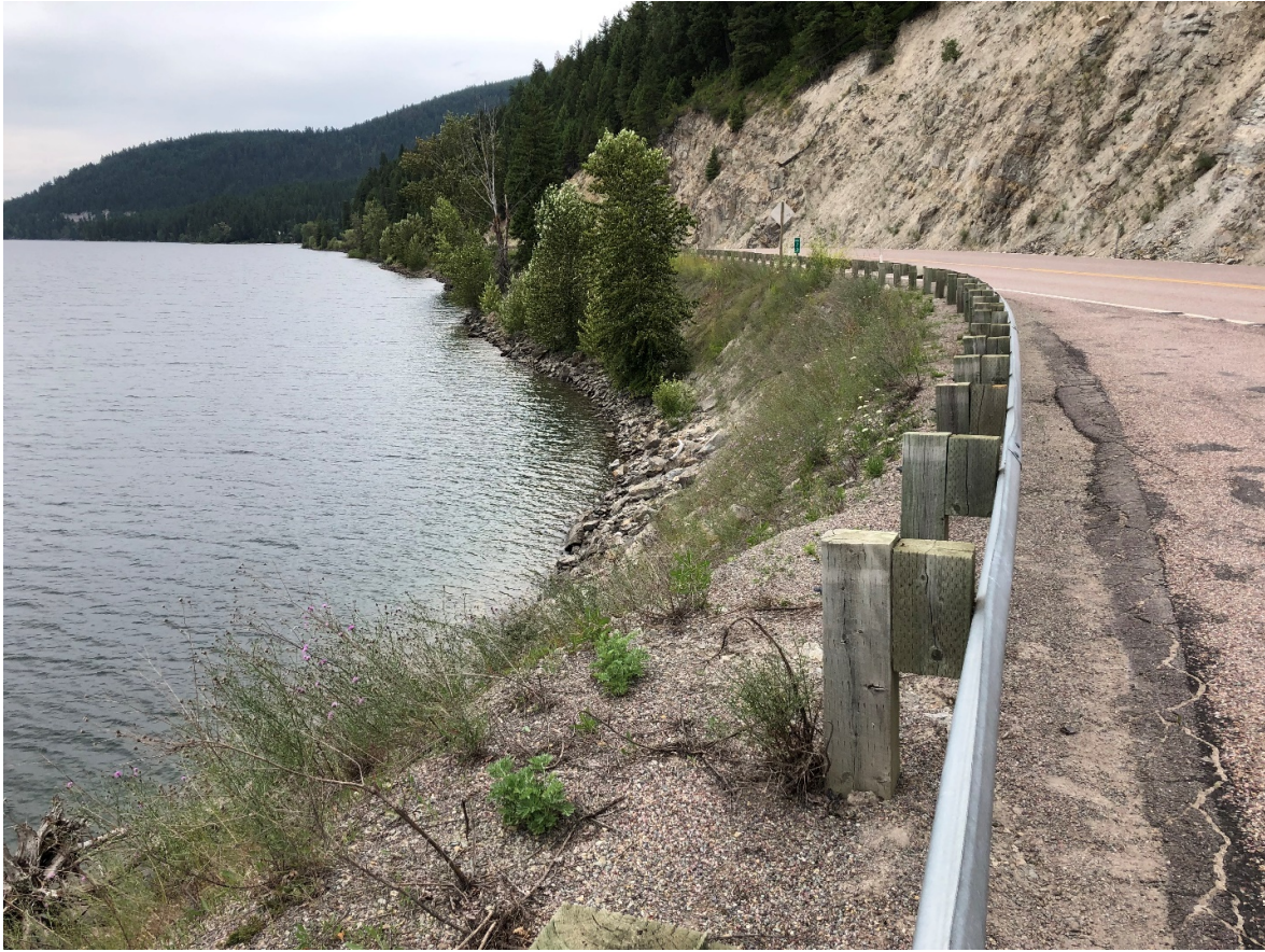
Figure 10 – Riprap protecting a highway embankment adjacent to a lake
