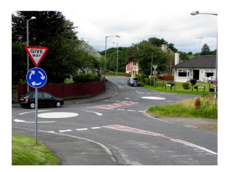
These changes improved the safety characteristics of the circular intersection by reducing the number and particularly the severity of collisions. Thus, the resultant modern roundabout is significantly different from the older style traffic circle both in how it operates and in how it is designed.
