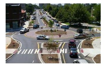
• The pedestrian refuge should be designed at street level, rather than elevation to the height of the splitter island. This eliminates the need for ramps within the refuge area which can be cumbersome for wheelchairs.
