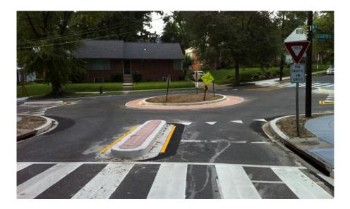
• *Roundabouts* are circular intersections with specific design and traffic control features. These features include yield control of all entering traffic, channelized approaches and appropriate geometric curvature to ensure that travel speeds on the circulatory roadway are typically less that 30 mph.
