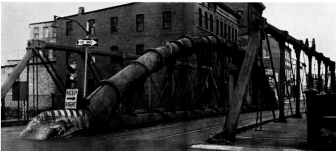
Figure 20.—Two views of Bollman-built “water-pipe truss” that carries Lombard Street over Jones Falls in Baltimore. Built in 1877.
