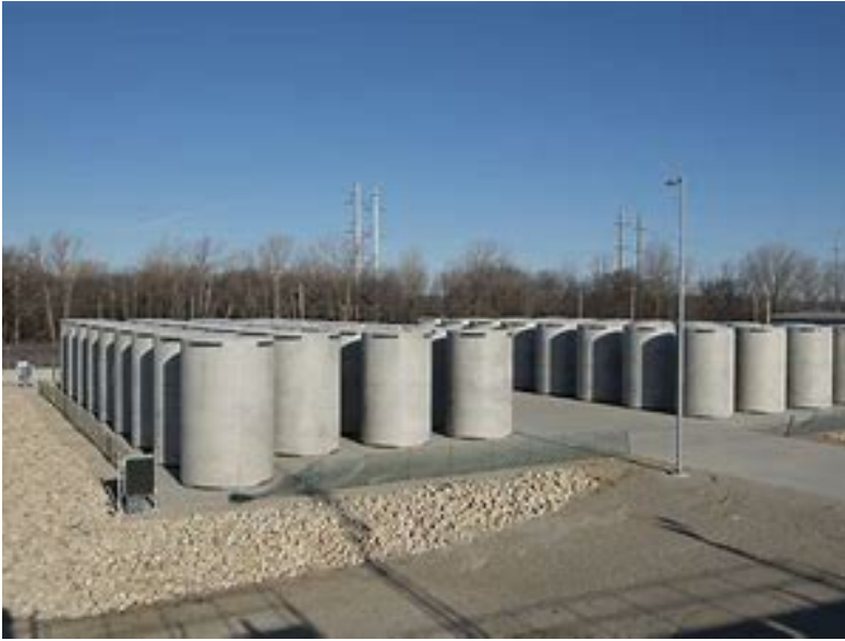
Figure 2-3: Example ISFSI at a Nuclear Power Plant 8
