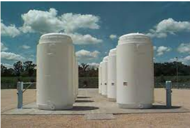
Figure 2-6: Bare Fuel Cask ISFSI
