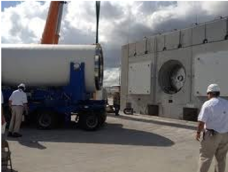
Figure 2-13: NUHOMS HSM Ready for Door Installation 17
