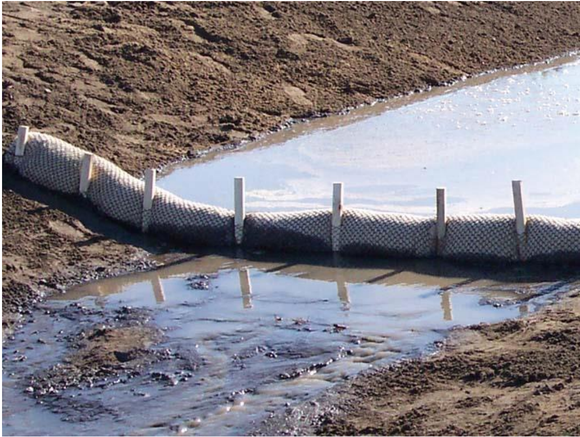
Figure 20 – Straw Logs Operated Effectively
