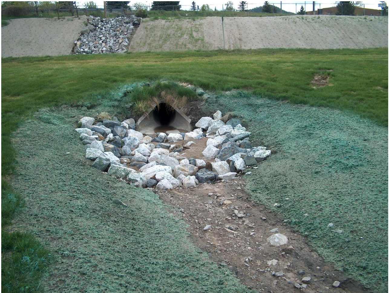
Figure 2 Riprap outlet protection and mulch/hydroseed along banks.
