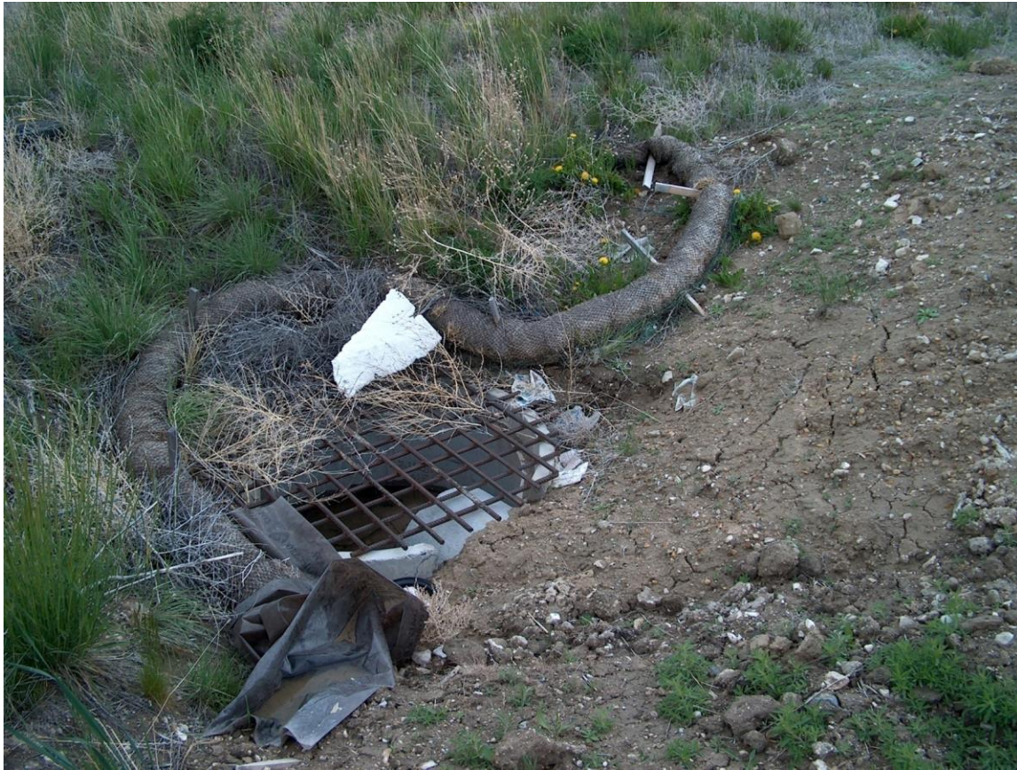
Figure 32 – Fiber roll around an inlet
