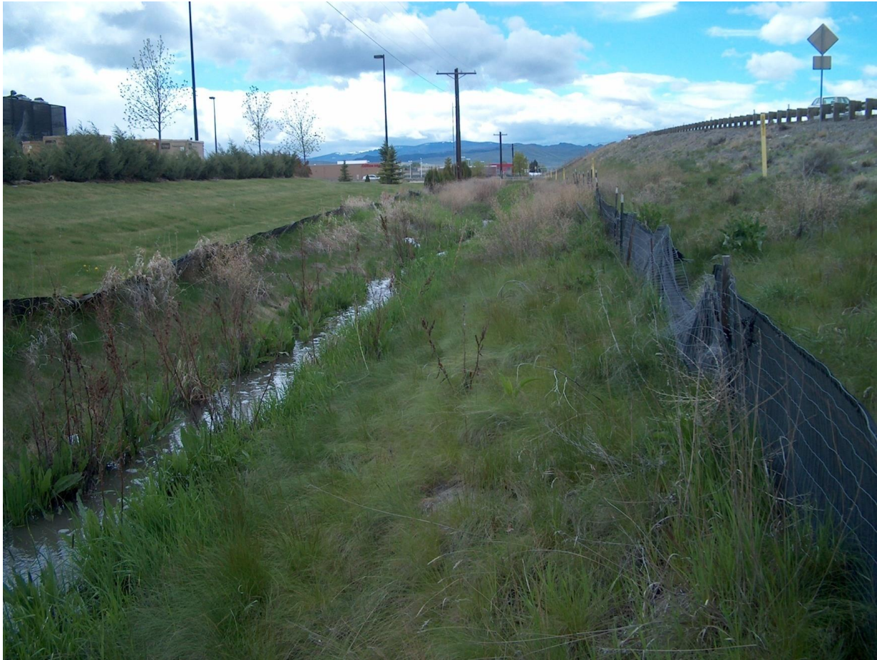
Figure 9 – Silt Fence after completed construction
