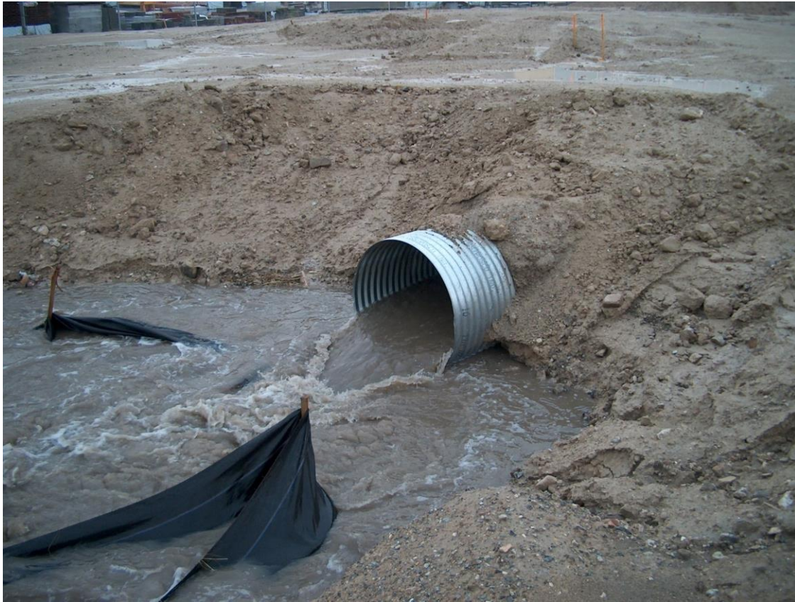
Figure 31 – Silt fence at the end of a culvert
