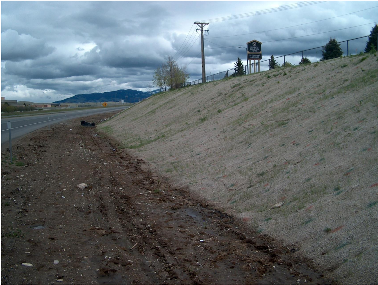
Figure 4 – Erosion Control Mat on a steep slope.
