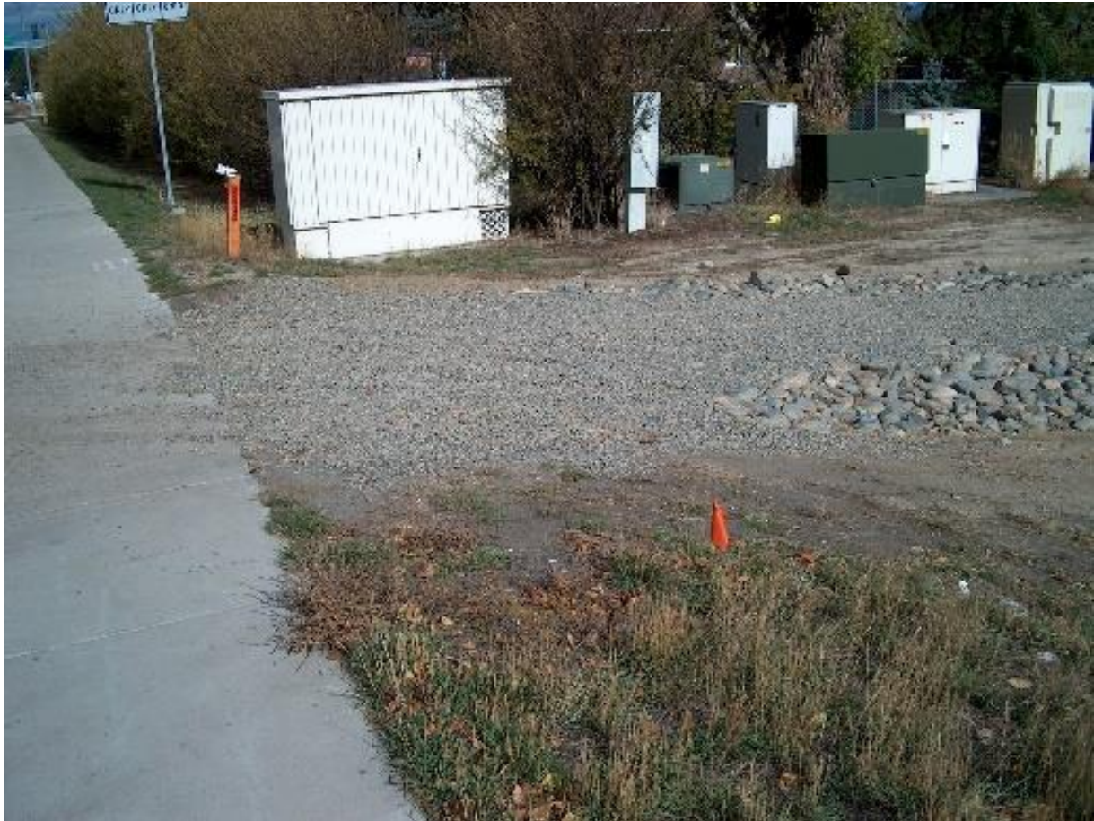
Figure 29 – Gravel Entrance at Roadway
