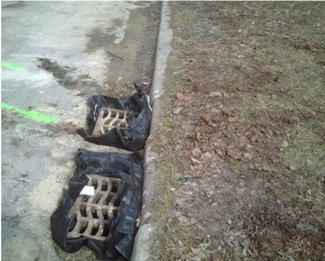
Figure 25 – Geotextile used as inlet inserts
