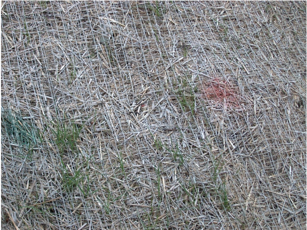
Figure 5 – Close-up of Erosion Control Mat with vegetation.
