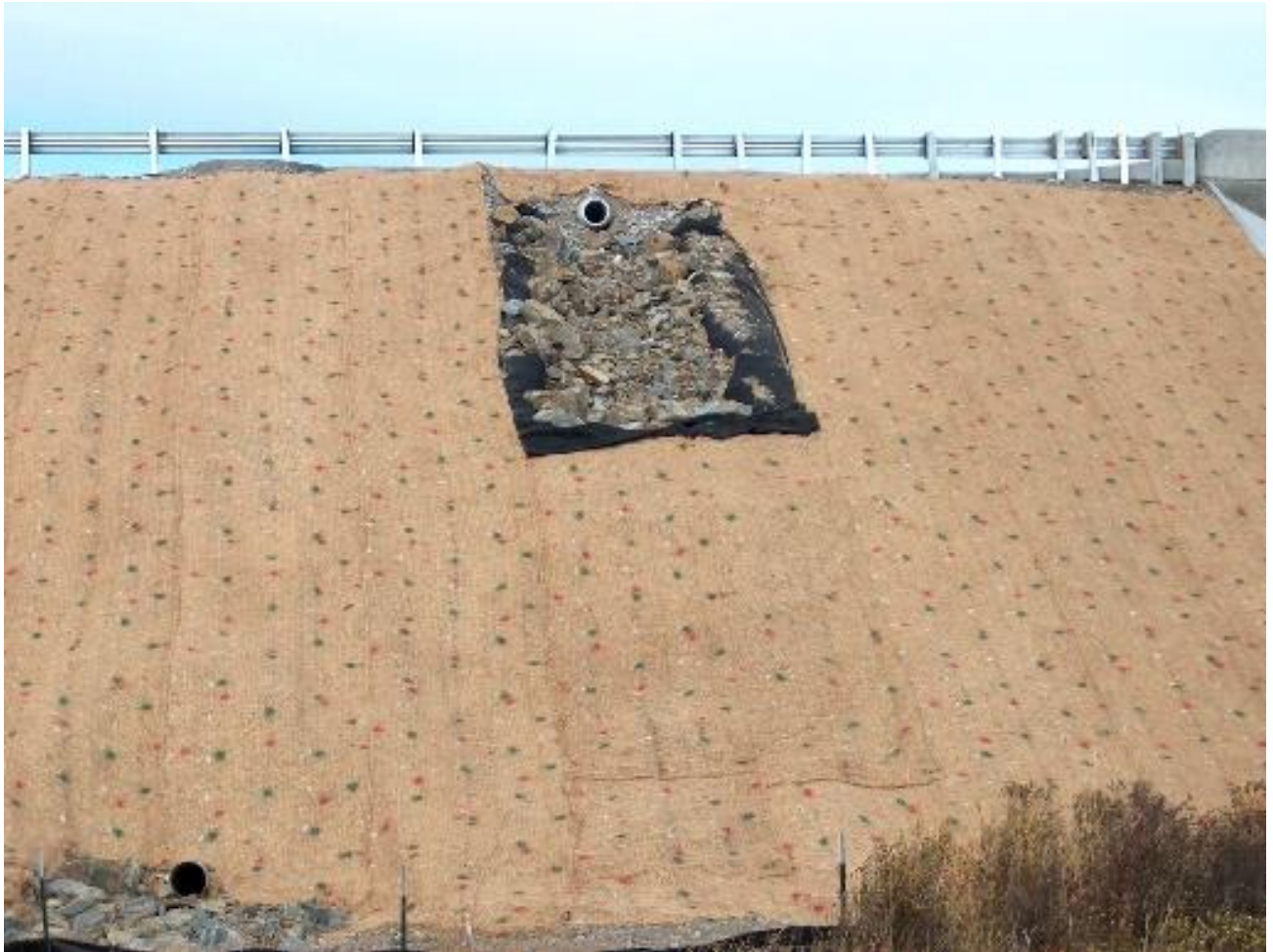
Figure 7 – Riprap and Erosion Control Blanket on Slope
