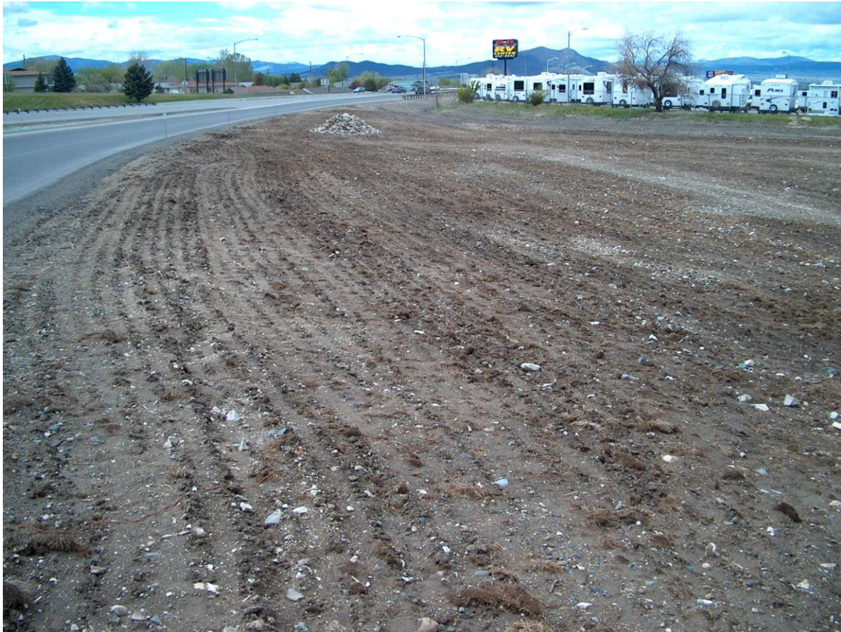
Figure 1 – Slope roughening
