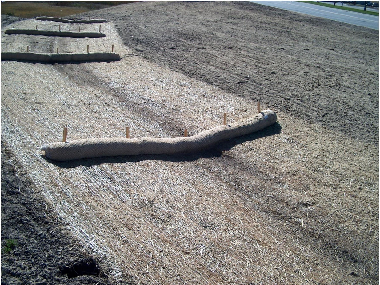
Figure 13 – Erosion Control Blanket and Straw Logs
