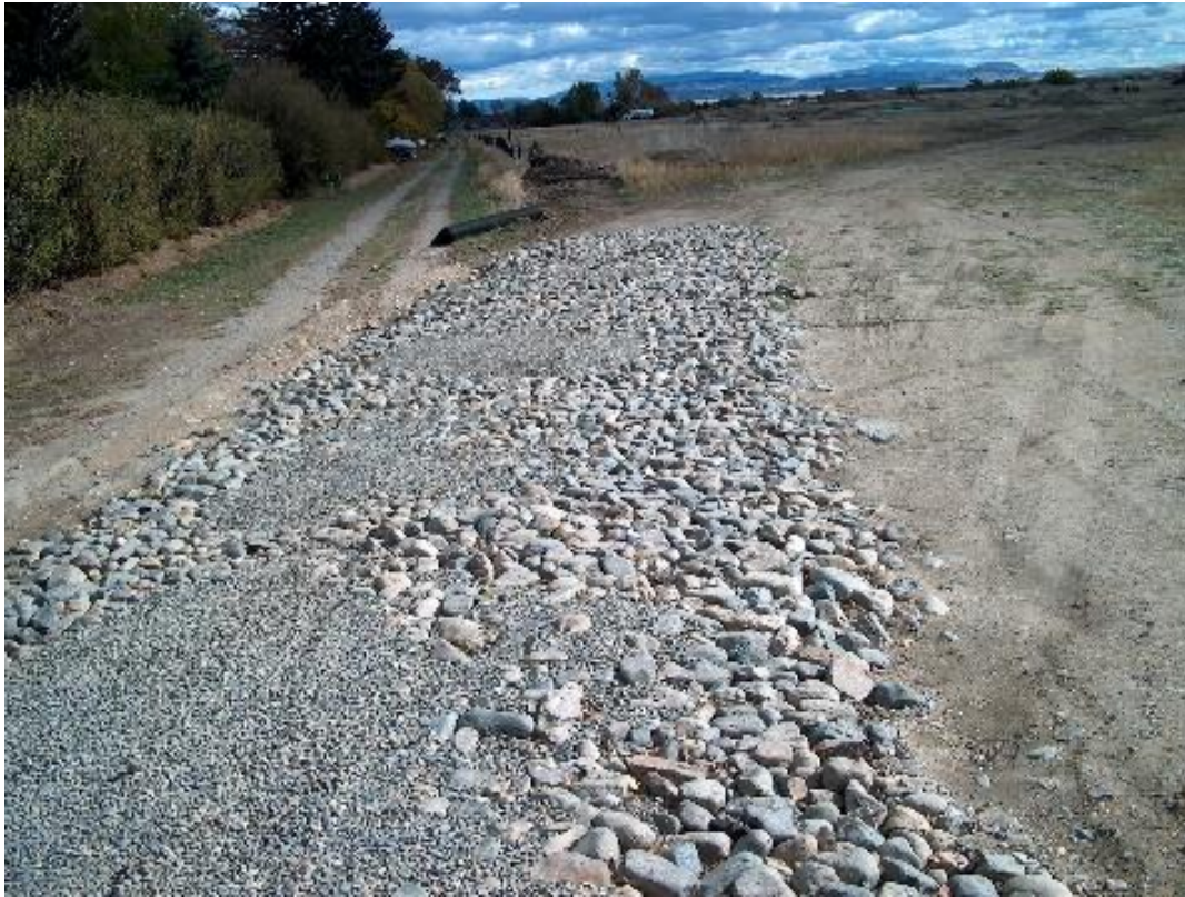
Figure 28 – Gravel Entrance at Disturbed Site
