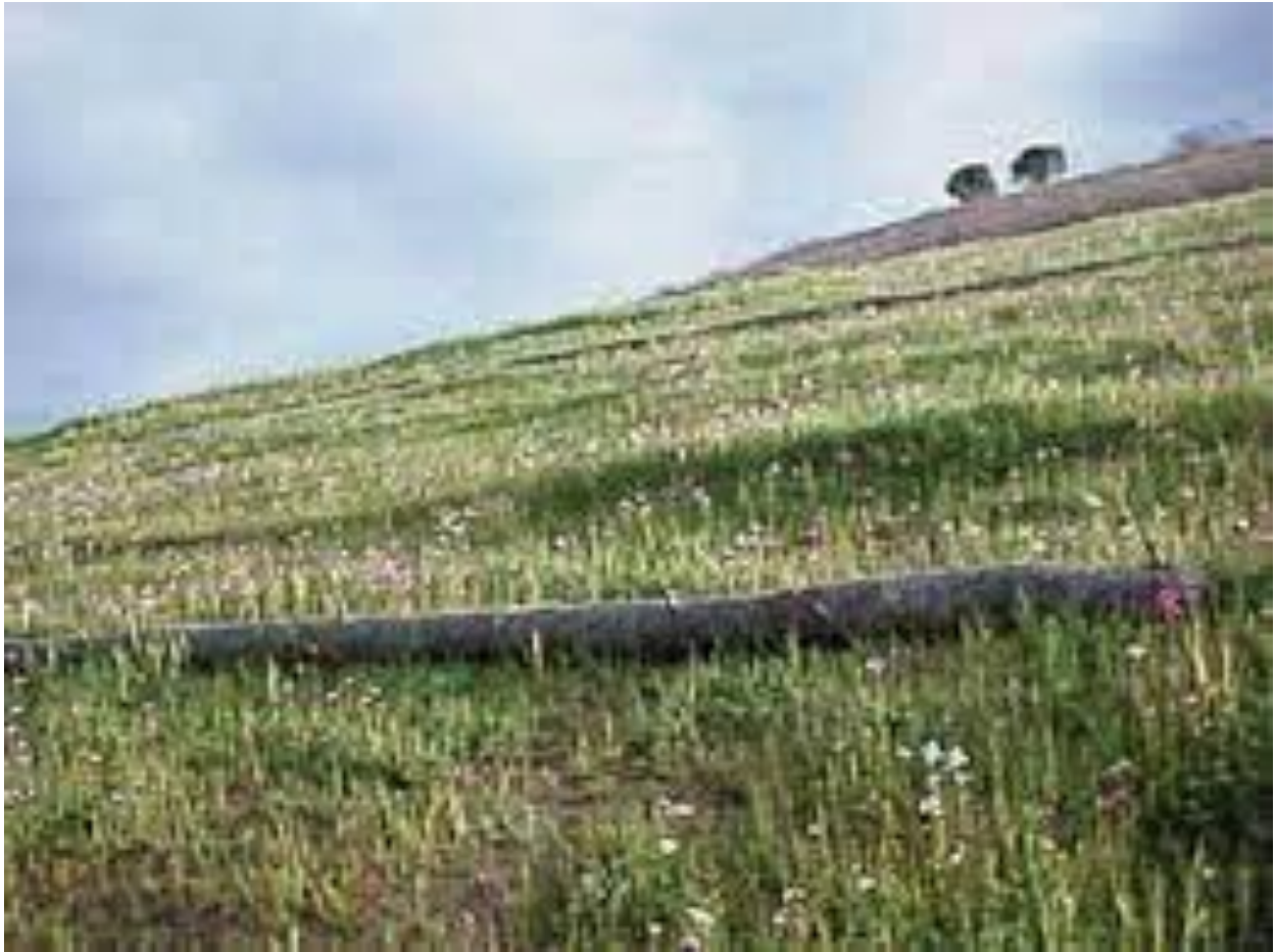
Figure 3 – Straw Logs on a Slope
