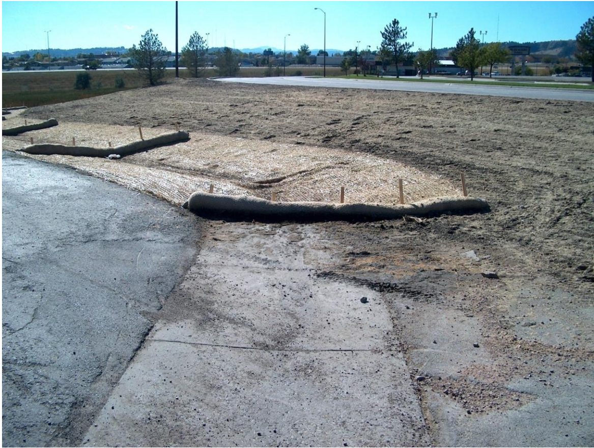
Figure 12 – Erosion Control Blankets and Straw Logs
