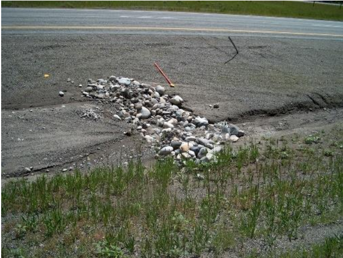
Figure 18 – Gravel Berm
