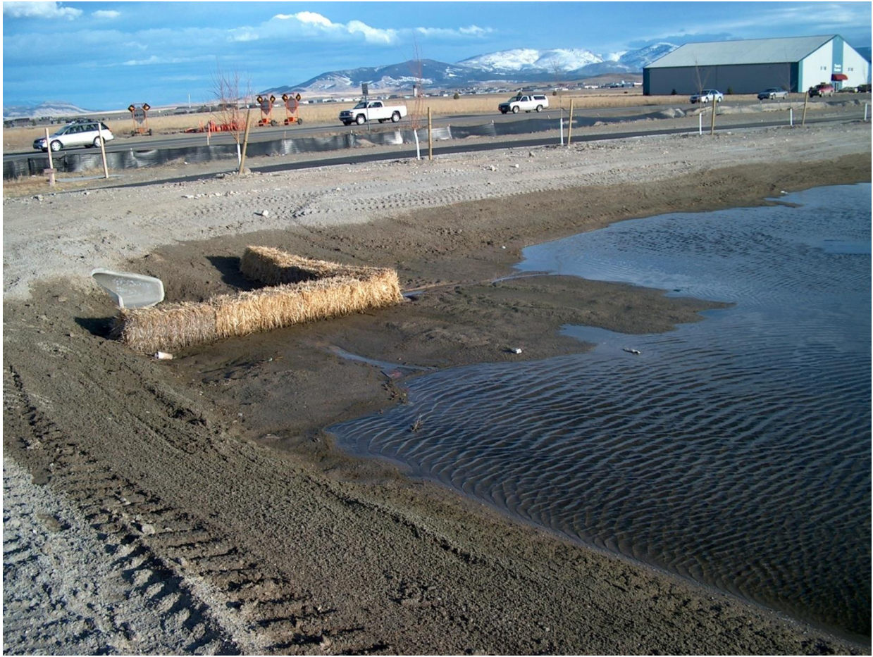
Figure 21 – Straw Bales used for Sediment Control
