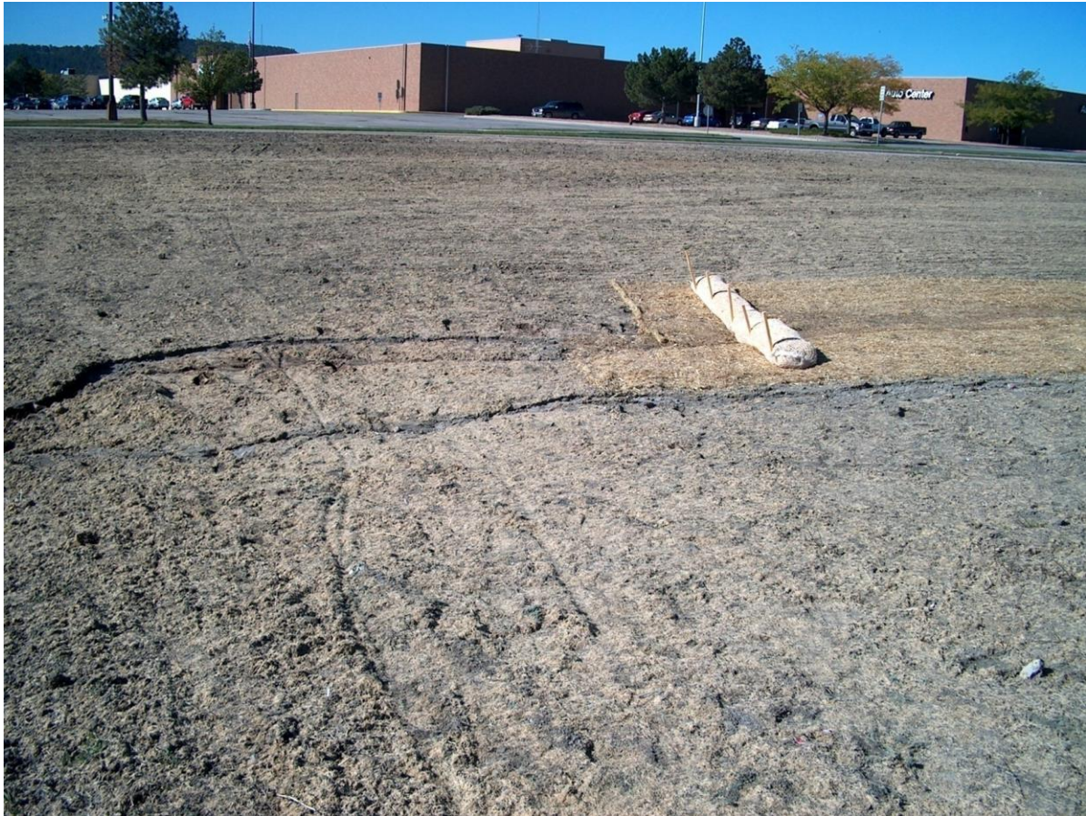
Figure 14 – End of Erosion Control Blanket
