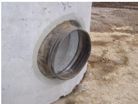
Figure 7 – Manhole Base Section with Rubber Boot
