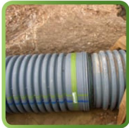
Bell/Spigot Joint Connection
