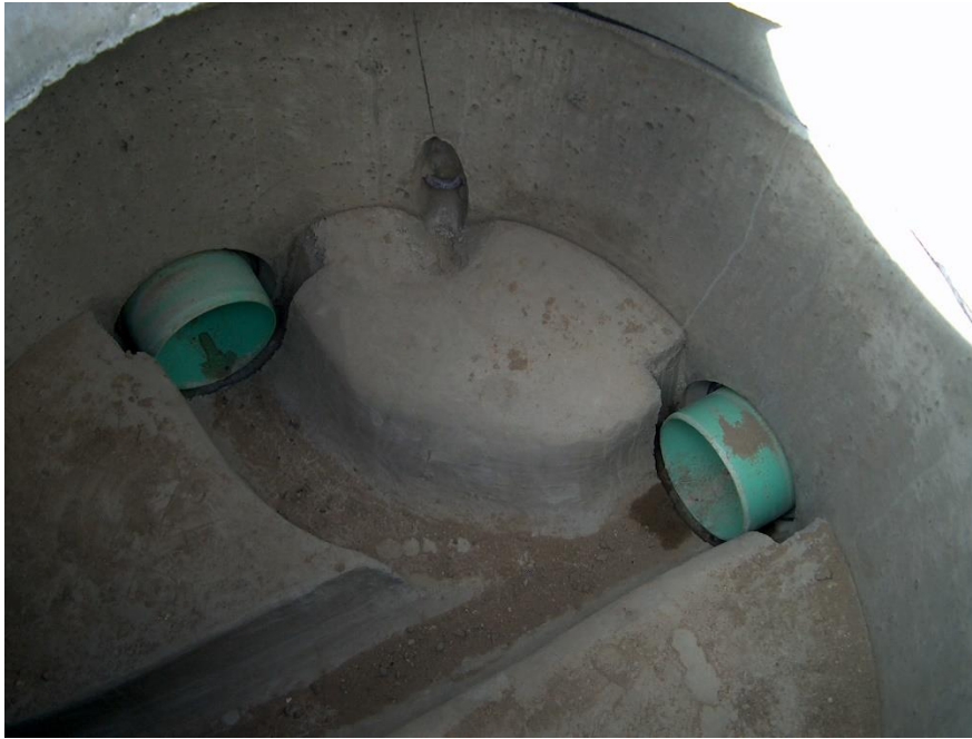
Figure 2 – Manhole Invert
