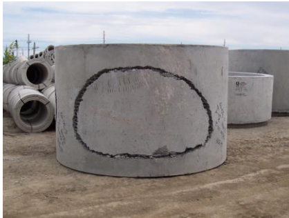
Figure 8 – Manhole Cutout for Large Diameter Arch Pipe
