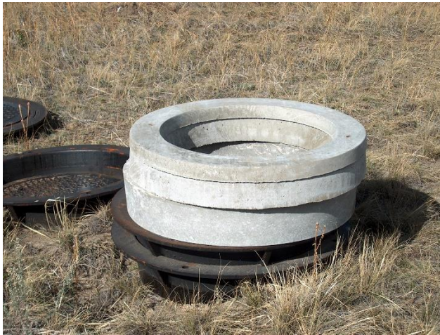
Figure 6 – Manhole Adjusting Rings
