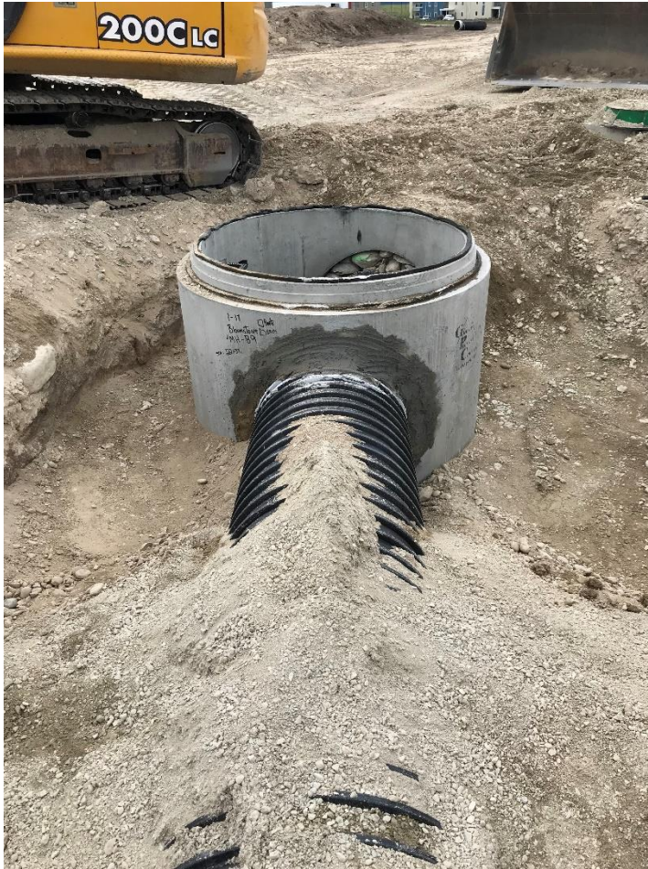
Figure 23 – Installed Steel Reinforced Corrugated HDPE
