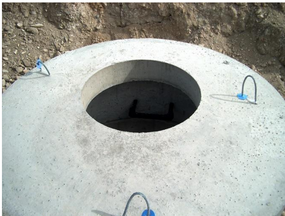
Figure 5 – Flat Slab Manhole Top
