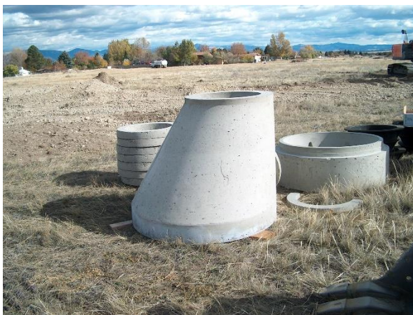
Figure 3 Eccentric Cone Section
