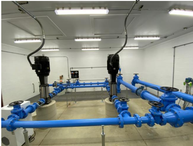
Figure 7 – In-line Vertical Turbine Pump
