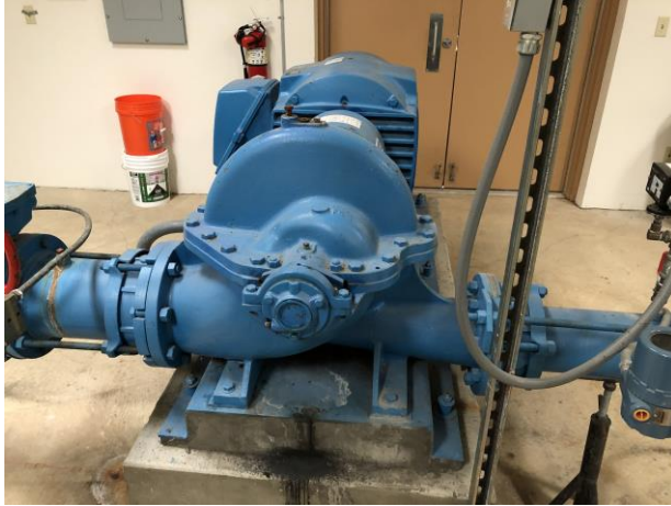
Figure 6 – Horizontal Split Case Pump
