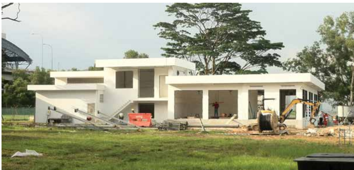
FIGURE 7.13 A substation under construction
