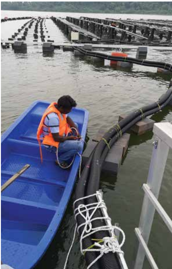
FIGURE 9.17 Maintenance on cables returning to shore
