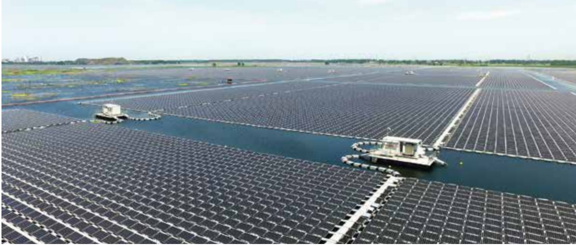
FIGURE 4.1 Central-inverter configuration for FPV systems, China
