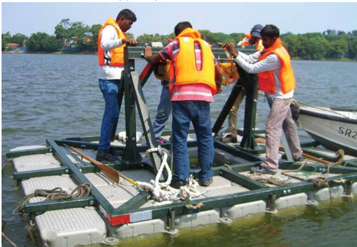
FIGURE 2.7 Concrete sinker test, Singapore Tengoh Reservoir testbed
