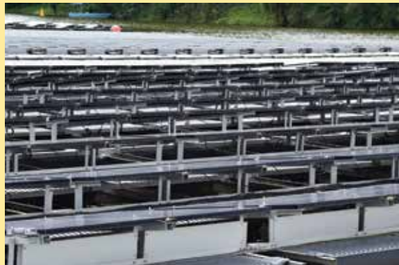
FIGURE 4.5 Windshields on the perimeter row of floats
