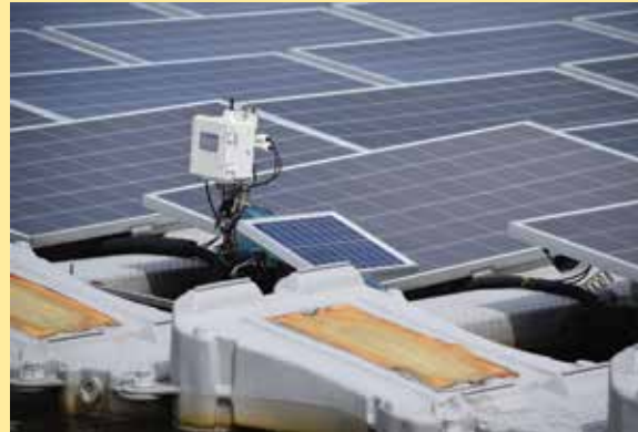
FIGURE 9.12 Sealing tape to cover open areas in floats
