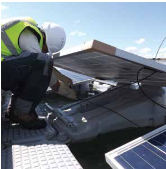
FIGURE 9.14 Corrective maintenance carried out on the float
