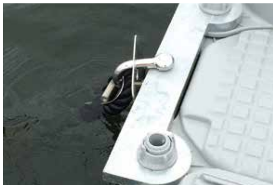
FIGURE 7.12 Mooring to the floating PV platform using D shackle with ropes (left) and using a spreader bar and chains (right)
