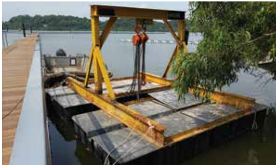
FIGURE 7.9 Barge used to lower concrete sinkers
