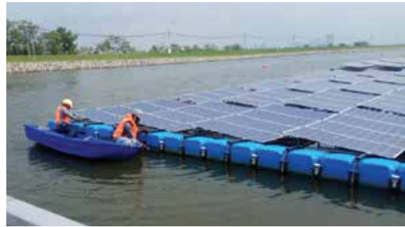
FIGURE 9.10 Floating islands constructed without walkways (left), and its maintenance (right)
