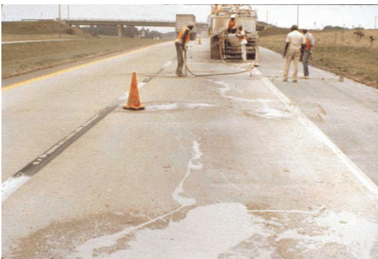
Figure 9-1. Fly ash grouts for pavement subsealing
