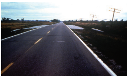
Figure 5-5. Bridge replaced by culverts and flowable fill.
