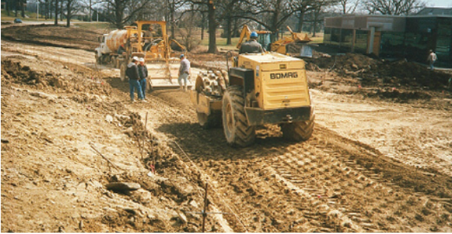
Figure 7-3. Mixing and compaction of fly ash into a plastic soil. Historically, plastic soils have been treated with quick lime ( \text{CaO} ) or hydrated lime [ \text{Ca}(\text{OH})_2 ] to lower their plasticity. The lime chemically reacts with the soil particles, effectively changing the soil grains from clay size (less than 0.002 mm) to silt size (0.05 to 0.002 mm). The determination of the plasticity index is geared towards measuring this chemical change in the soil.
