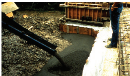
Figure 5-4. Bridge abutment backfill with flowable fill.
