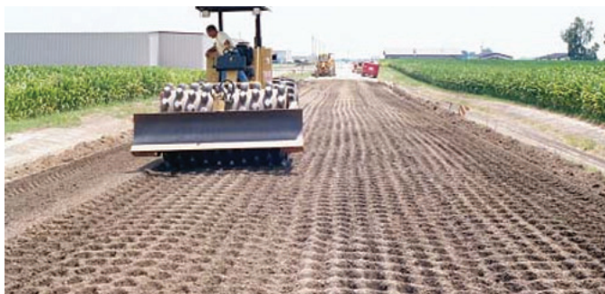
Figure 7-2. Compaction of fly ash stabilized soil.
