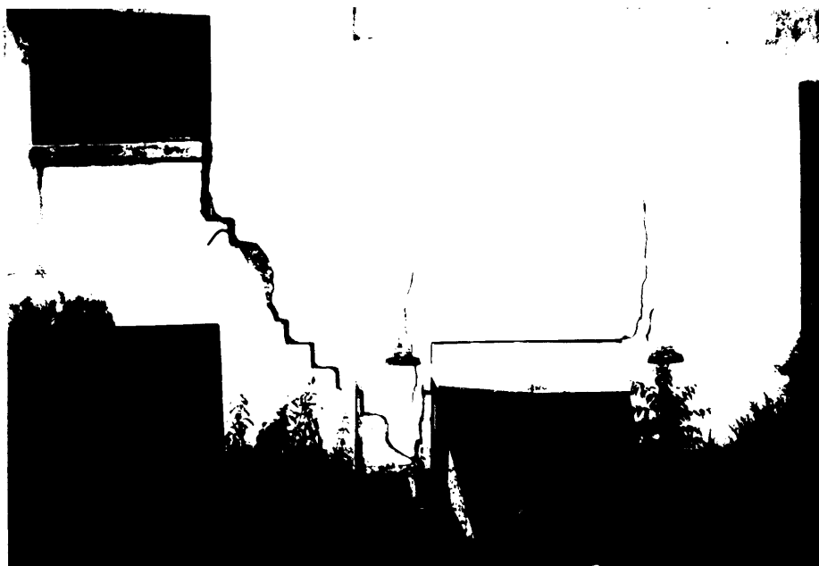
b. Diagonal and vertical cracks
