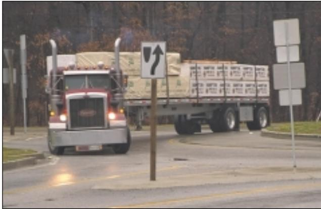
Good roundabout design makes accommodation for the appropriate design vehicle. For small roundabouts, this may require the use of an apron. *Lothian, MD*
