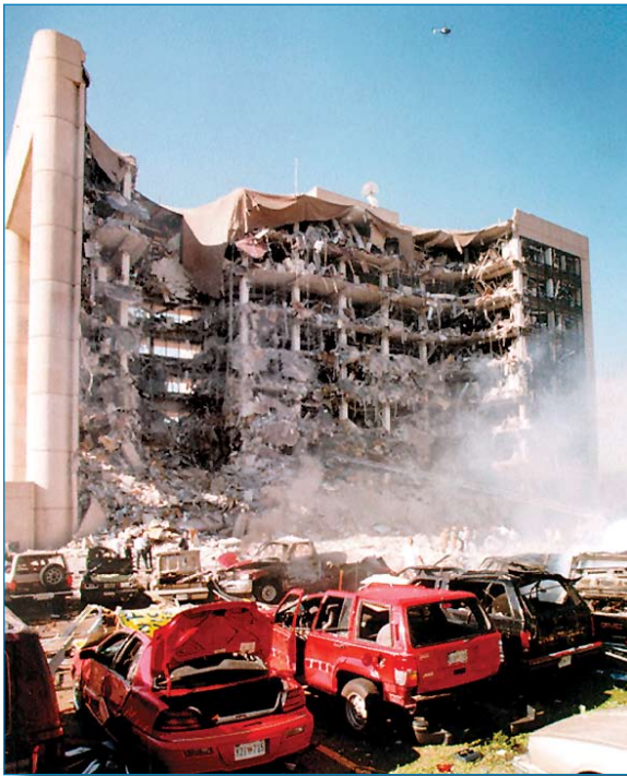
Figure 2-4 Alfred P. Murrah Federal Office Building
