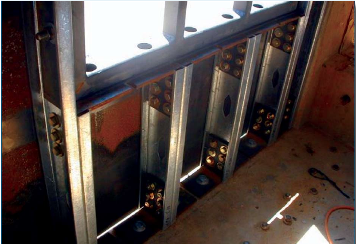
Figure 2-19 Metal stud blast wall
