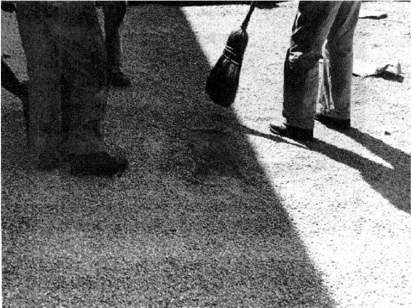
Figure 11. Insufficient bitumen to embed aggregate surfacing.
