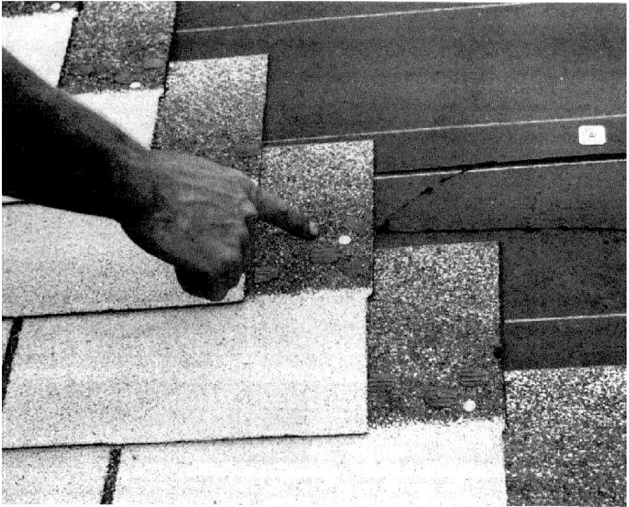
Figure 4. Asphalt shingles nailed too high.
