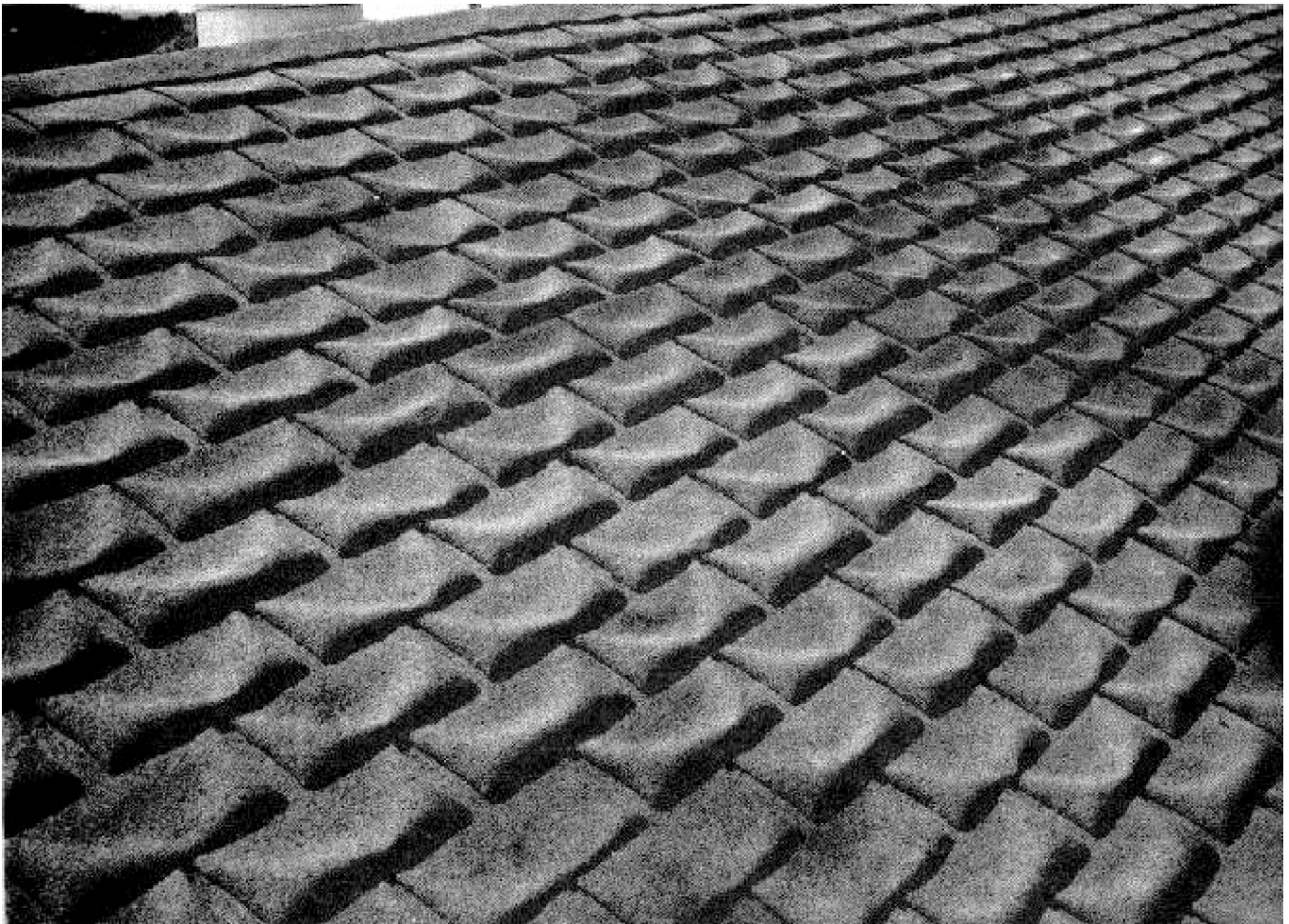
Figure 26. Clawed asphalt strip shingles.
