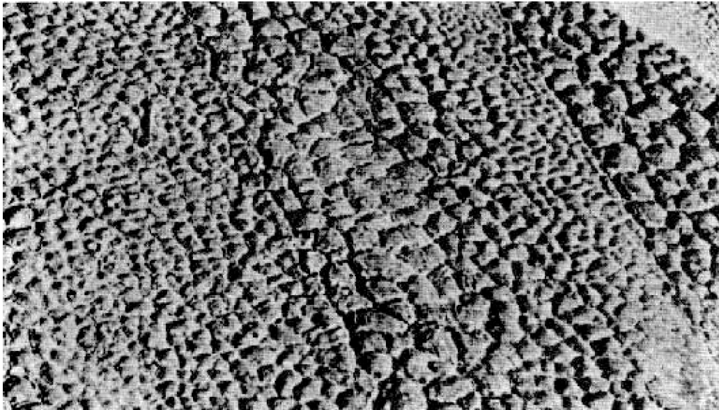
Figure 17. Alligating and cracking of a cold coating over alligatored asphalt surface after 1 year exposure.
