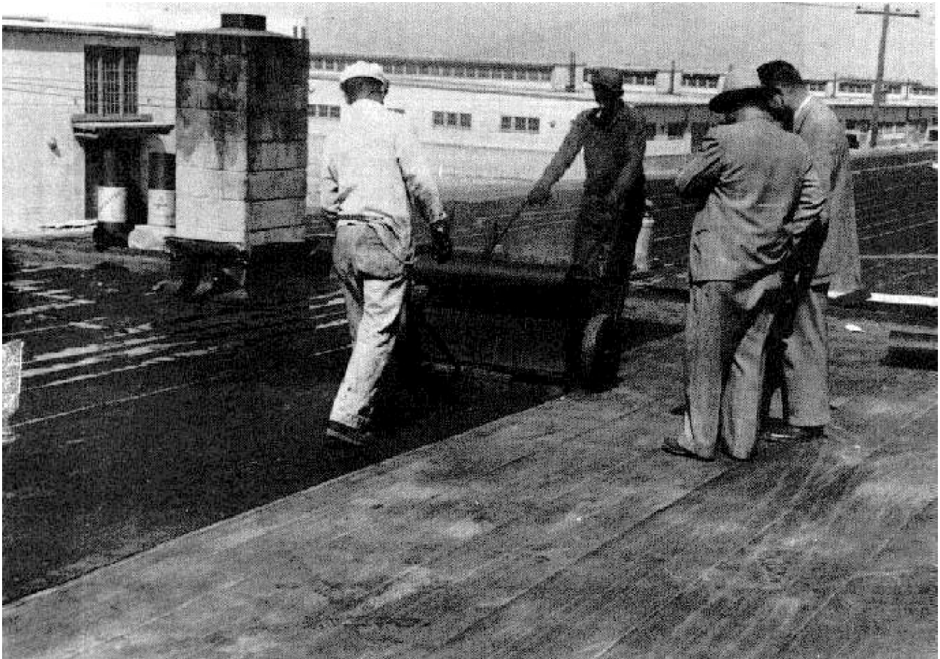
Figure 9. Laying felts mechanically and brooming-in after felt is rolled into hot bitumen.
