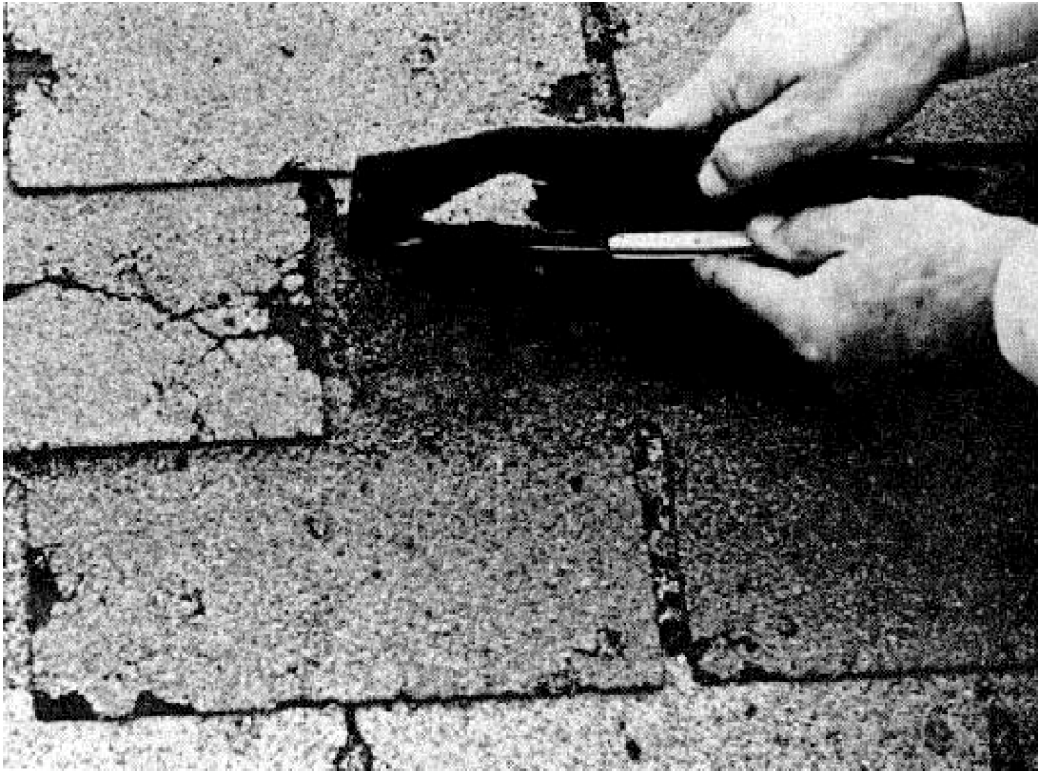
Figure 30. Hail damage showing broken shingles — reroofing mandatory.
