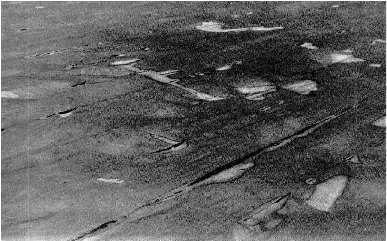
Figure 3. Wrinkles, buckles, lack of adhesion of felts.
