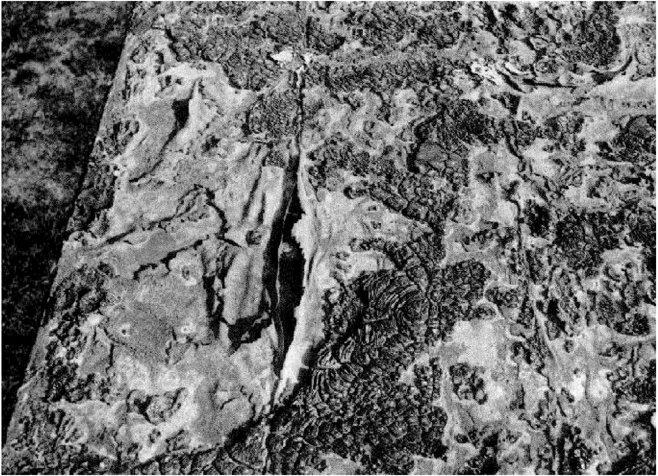
Figure 20. Felts disintegrated and disbonded – reroofing is mandatory.
